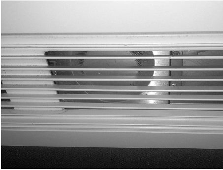
Fig. 14. Installation in the air duct
