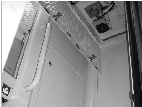
Fig. 16. Installation in a toilet
