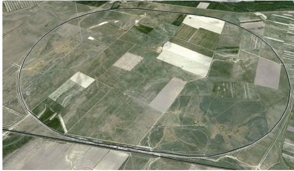
Fig. 7. Faurei Railway Testing Center
