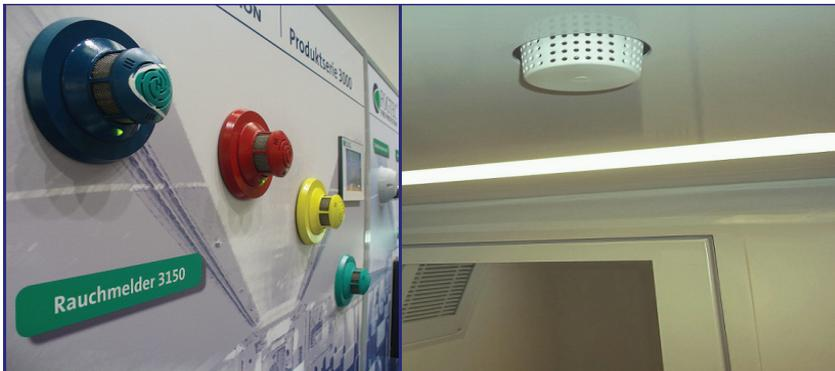
Fig. 5. Examples of different detectors and application in a EMU’s vestibule [2]
